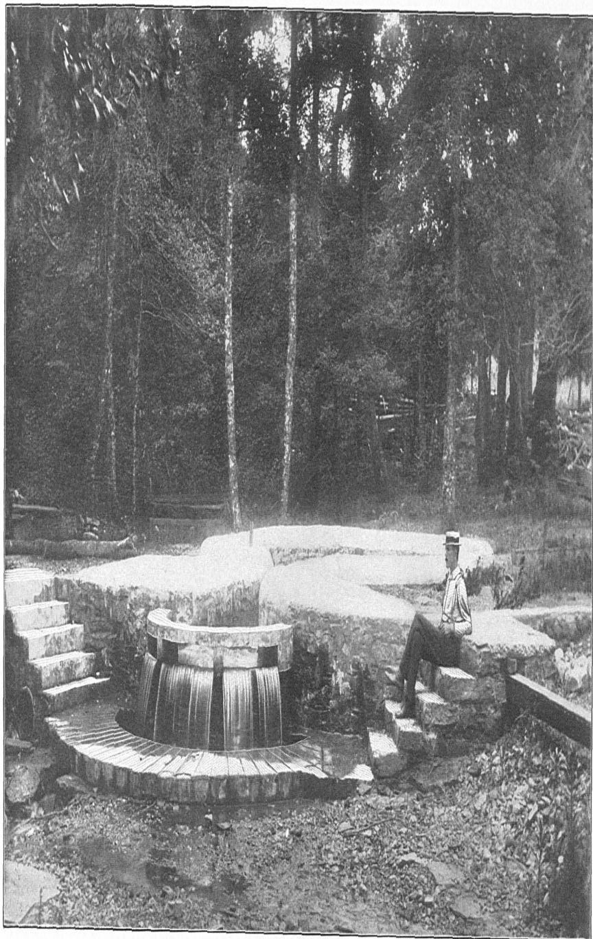
COLD SPRING—PART OF WATER SUPPLY AT BULLOCHVILLE.
