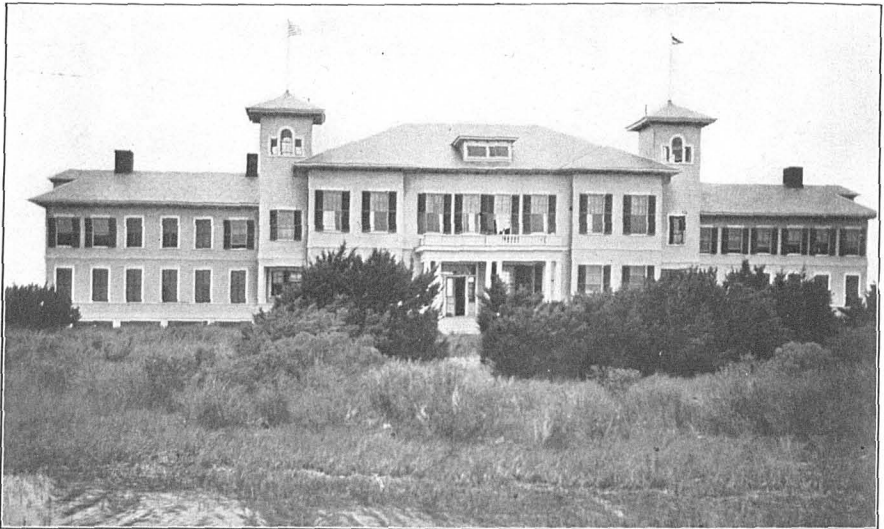
BEAUFORT LABORATORY—EXTERIOR VIEW.
