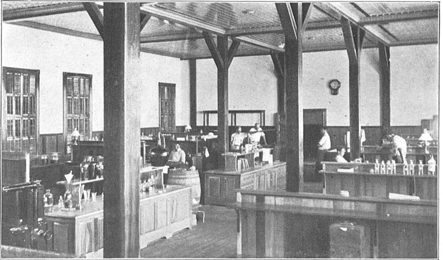
LABORATORY INTERIOR, BEAUFORT.
